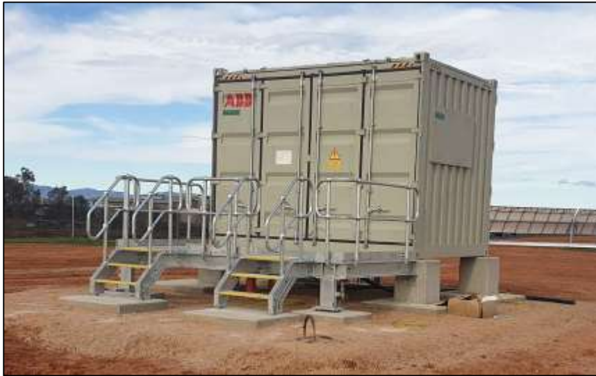
Figure 5 – typical HV Switchboard (Source: Green Gold Energy)
